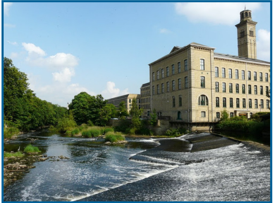
Salts Mill and River Aire, Saltaire
