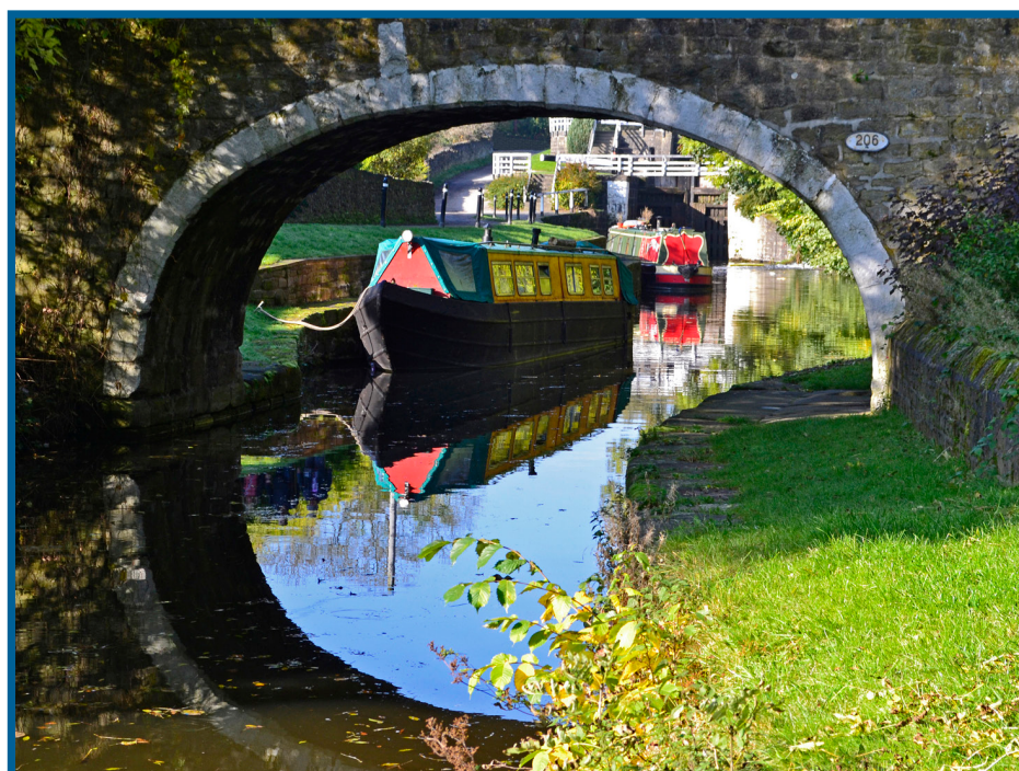
Dowley Gap, Leeds Liverpool Canal, Bingley
