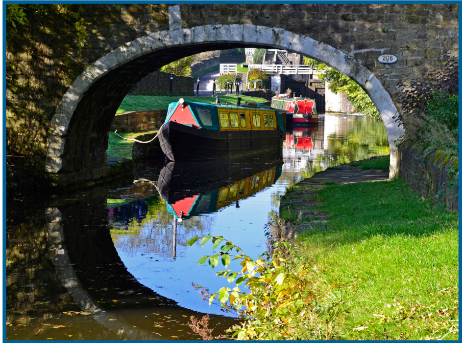
Dowley Gap, Leeds Liverpool Canal, Bingley
