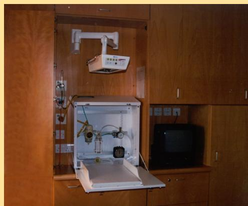
Cabinets are available in a variety of configurations suited to individual requirements. The pictures to the right depict a cabinet configuration which has a Tom Thumb unit without an integral flow meter, so as to be used with an existing external flow meter.
