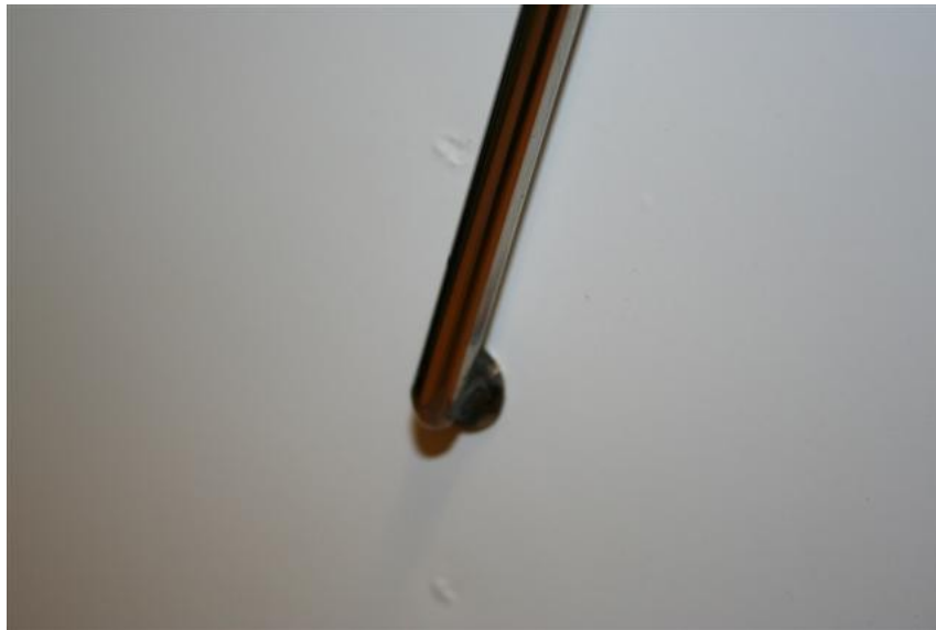
fig.3 (Spot-welding marks above and below the hinge)
