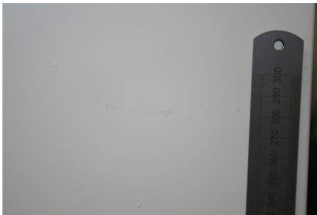
fig.2 (Paint blemishes running horizontally)
