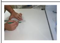
Open the door on the Resuscitation Cabinet and using a rule, mark a cross in the centre point of the platform. The lines of the cross should extend to each side of the platform.
