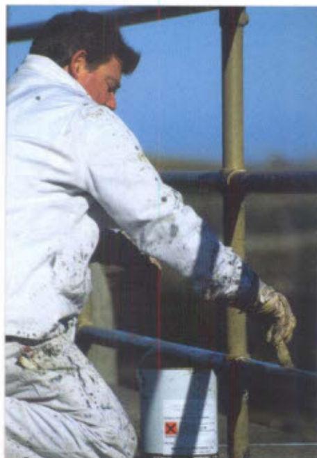
Overalls and gloves are needed to control the painter's exposure to this weatherproofing paint which is labelled with the hazard symbol for an irritant or harmful substance.
