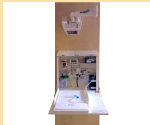
Infant Resuscitation Cabinet system shown mounted on wall strengthening pattress board
